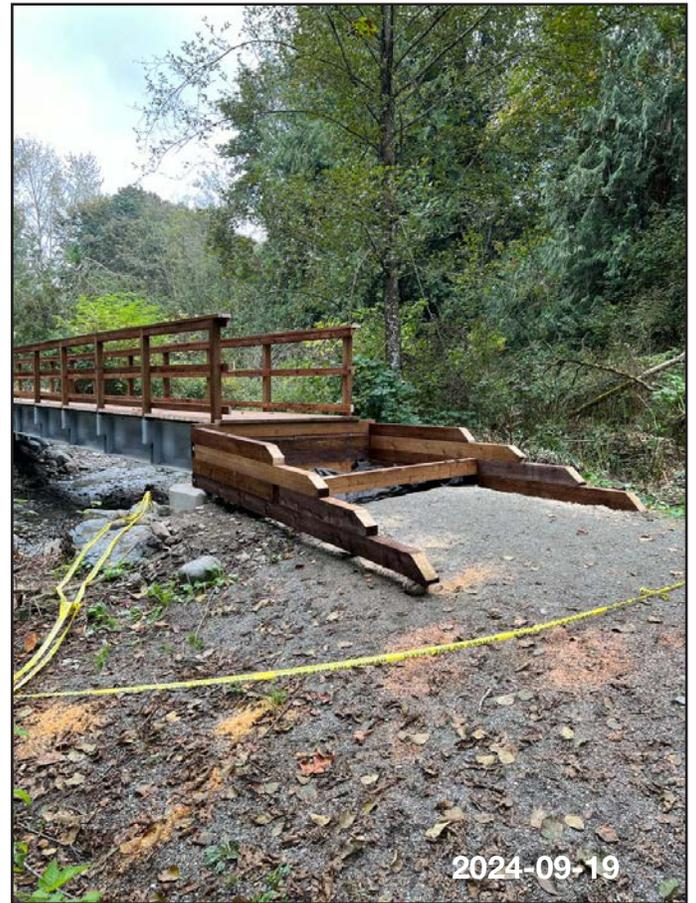
**Above:** the woodwork included a frame to retain a gravel ramp at the north end. **Below:** at the south end, boulders were used instead of a wood frame. While the Bridge was being assembled, machine operators were spreading new gravel and building up the path south of the Bridge.
