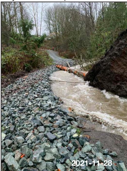
Then, at the end of that month, the second stage of the Atmospheric River dropped another 162 mm of rain. This time, the water in the secondary channel took out the old bridge completely and toppled the larger of the two cedars (that dark shape on the right of this photo is the huge mass of soil held by its roots).
